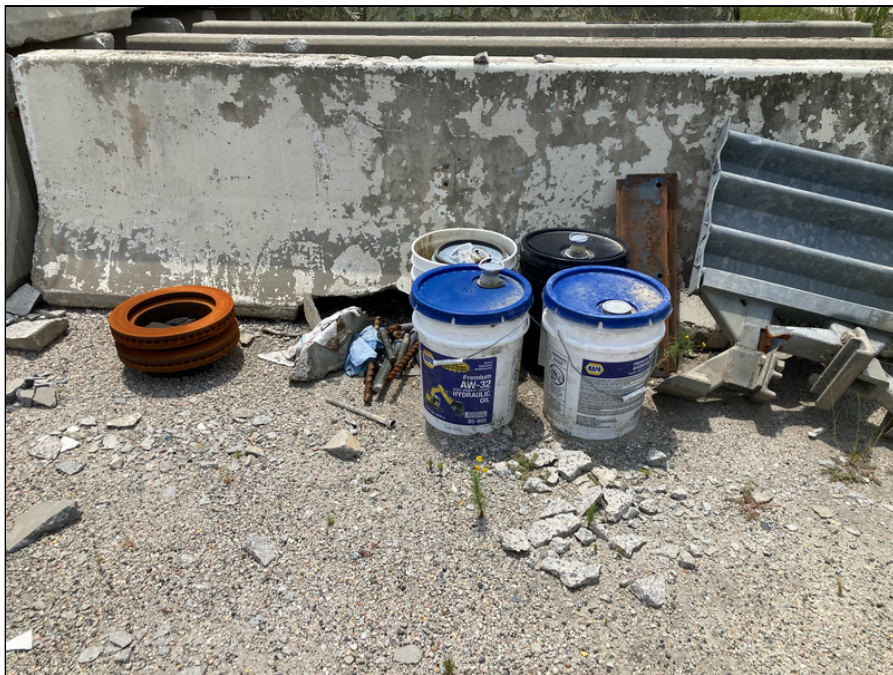
12 - View of the containers of hydraulic oil and motor oil.
