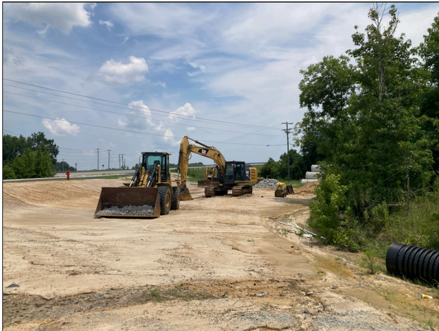
20 - View of the eastern adjacent construction site.
