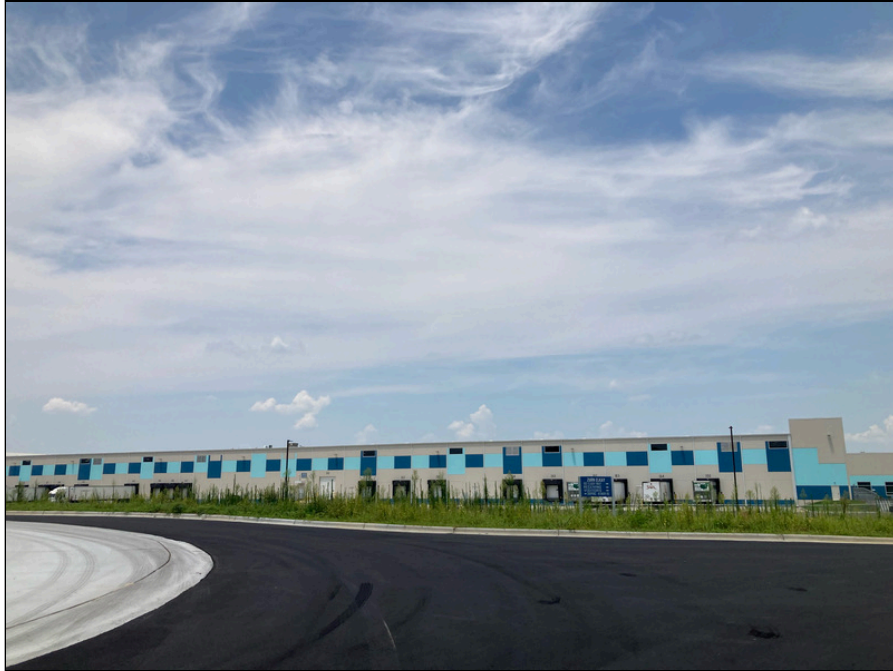
19 - View of the northern adjacent commercial building.
