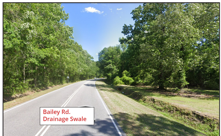
Existing Drainage System (Bailey Road)
