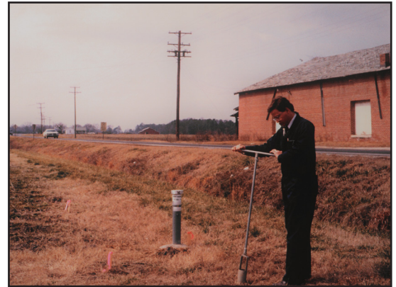
Founder Rick Catlin utilizing a hand auger to sample soils in 1990s.
