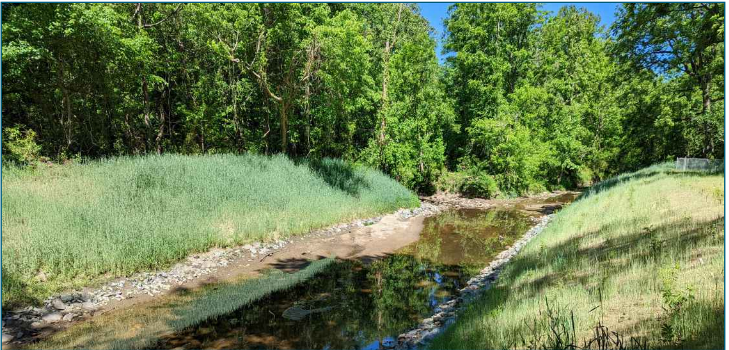
Emergency Watershed Protection Streambank Stabilization, Durham, NC
