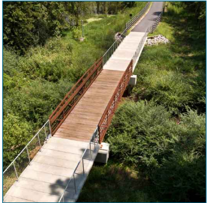
Smith and Sanford Creek Greenway Pedestrian Bridge, Wake Forest, NC
