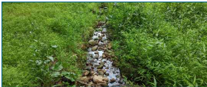
Ailey Young Dam Removal and Stream Restoration
