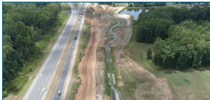
Smith Creek Relocation, Kernersville, NC
