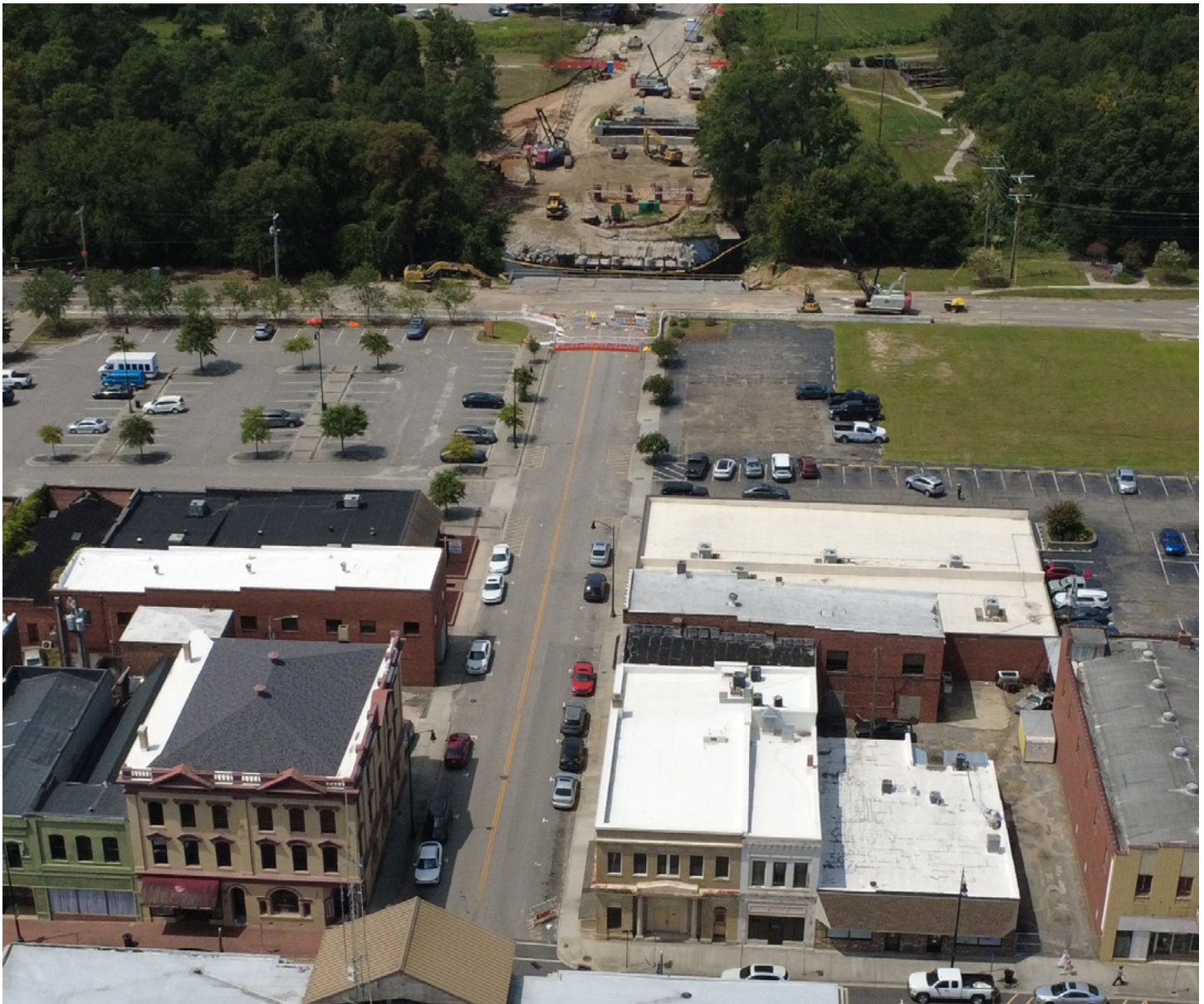
▲ View of Water Street and the 5th Street Bridge Replacement across the Lumber River.
