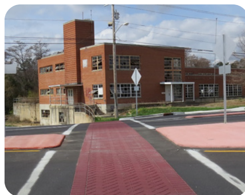
Water Treatment Plant
